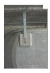
7. Repeat steps 4-6 being sure that the skirt is vertical AND the apron is even/level across the horizontal/long side of the skirt. Repeat steps 4-6 one more time until a total of 3 support brackets are attached to the skirted bathtub.
